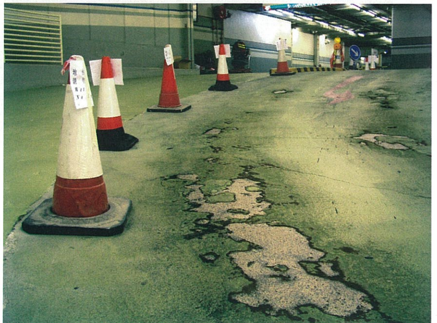
Typical PU flooring failure in Hong Kong where the resilience of the PU coating is no match for the rubber tires.
