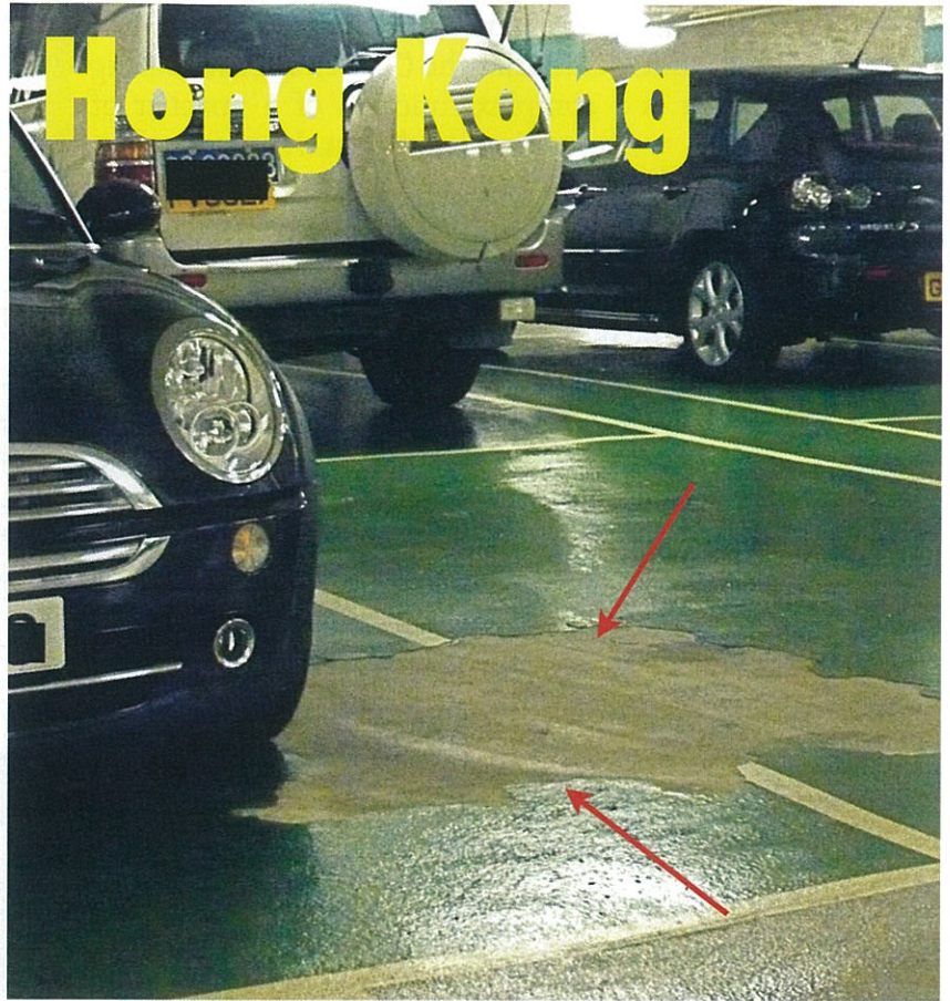
Typical PU flooring failure in Hong Kong where the resilience of the PU coating is no match for the rubber tires.
