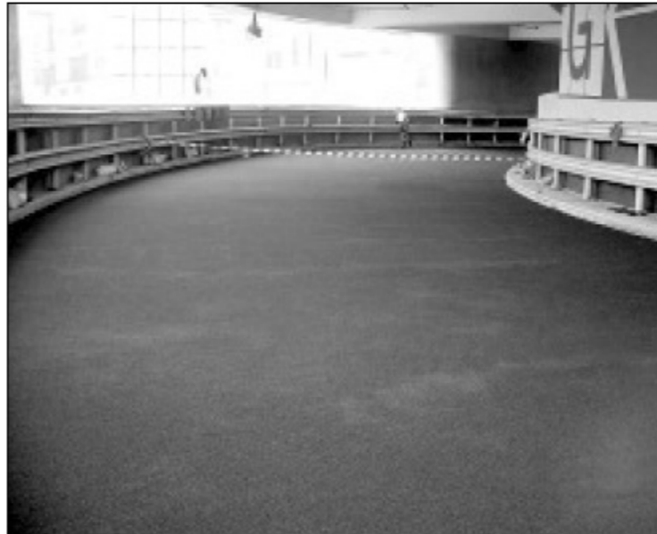
Cicol ET Slurry Application at a carpark in Hong Kong
